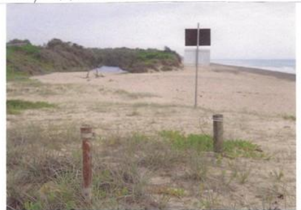
2007 - 17 years after the Gabion Wall was built.
