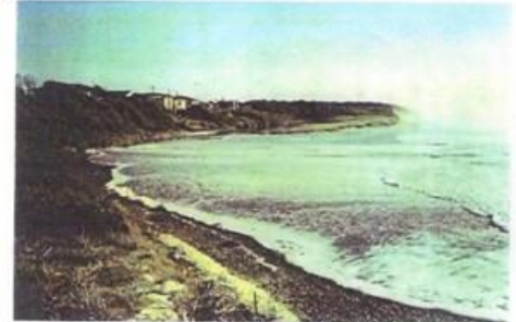
1989 - Before Erection of Gabion Wall
